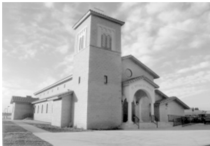
Taken from the side, and with a 40 yard dumpster still in view, one gets the idea of the size of the new church.
