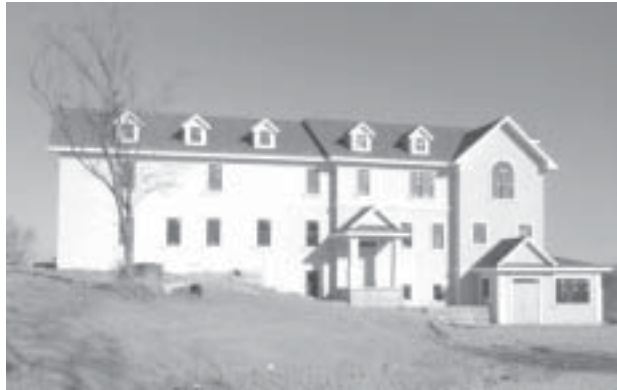
The new Regina Coeli House, shown after the windows and exterior doors were installed.
