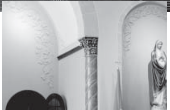
...marbleized columns, a simulated stone arch, and stenciled grape and leaf patterns on the inside walls of the arches.
