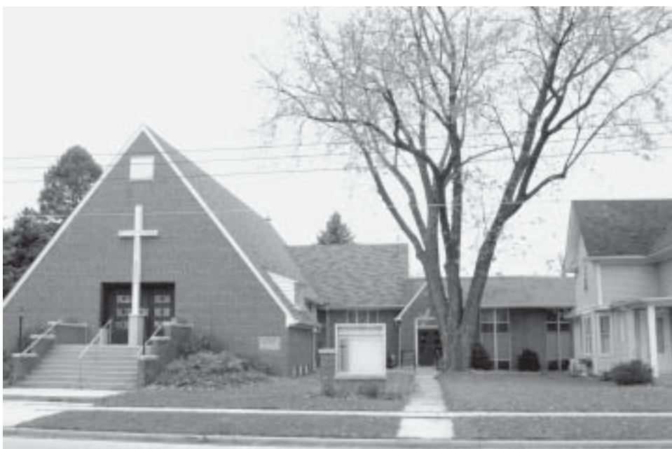
A view of the new additions to the parish complex.
