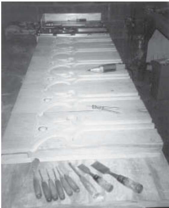
The mission caretaker has undertaken the construction of a new communion rail, properly imitating the frontal of the altar. Here, sections cut from custom stainless steel templates await the time-consuming carving only the human hand can do.
