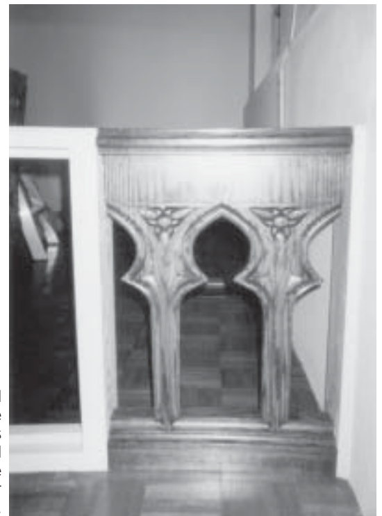
A finished section of the new rail has been installed next to the current one for display.
