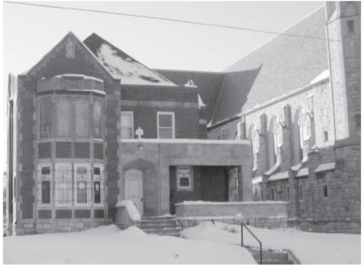
The Vincentian rectory, that now serves as the parish office, bookstore, classrooms, workshop and living quarters for lay workers, as the priests reside at the Regina Coeli House.
