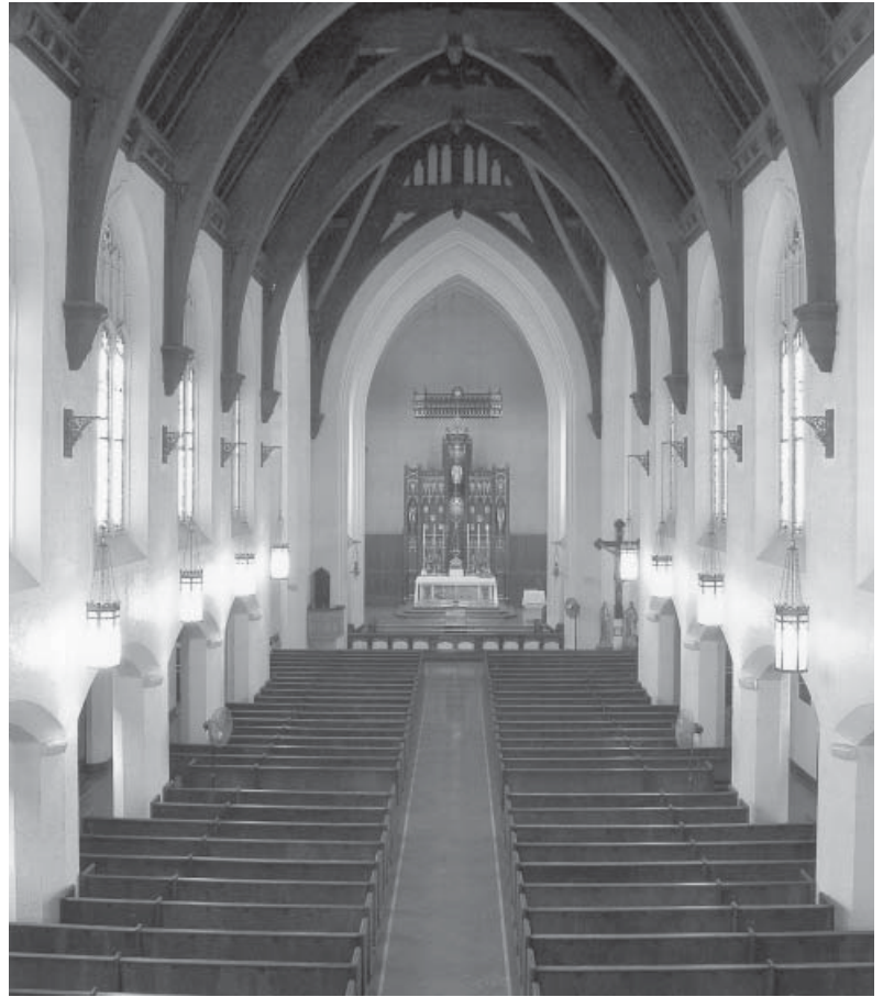
Cloister-style arcades and a nave directing focus to the high altar endow St. Vincent's with the contemplative qualities of a monastery chapel, while retaining enough decoration for a parish church. The church is 193 feet long and its interior apex, supported by gothic rafters of California redwood, is 69 feet high.
