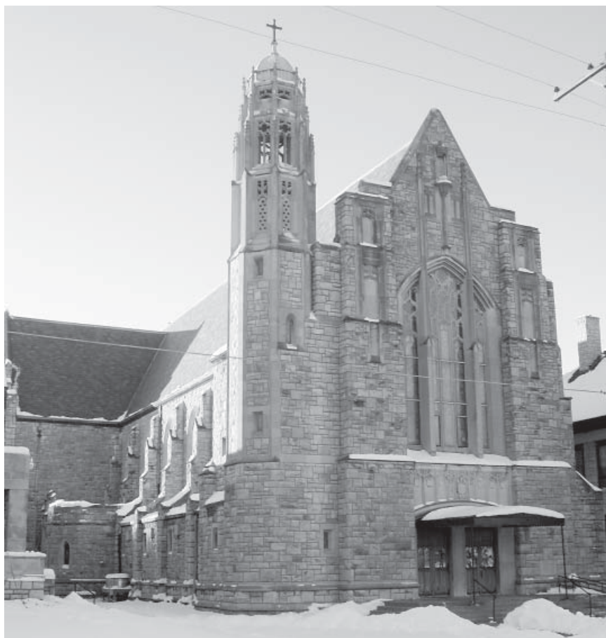
The church's unique façade, complete with blind niches (a common feature on English churches) that flank the choir window. Inside the copper-domed tower is the cathedral's former bell, large and sonorous, that Fr. Bernard Donnelly (1807-80; Kansas City's "pioneer priest") had cast for his first church. Put in the cathedral, then taken down in 1895, Bishop Lillis gave it to the new St. Vincent's.
