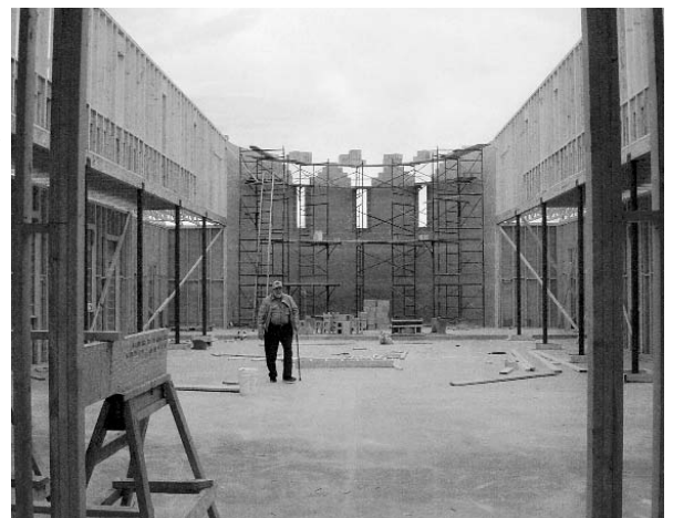
An inside view of the continuing wood framing and masonry construction.
