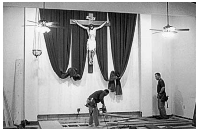
A shot of the beginning stages of the remodeling process. The single step has been removed in preparation for the addition of the new three stepped predella.
