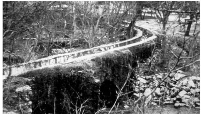
A partial view of the still-working stone aqueduct situated not far from the Mission San Jose. The Spanish missionaries built an interconnecting system of acequias (a network of gravity-flow ditches whose use originated in Moorish Spain), aqueduct and 5 dams covering 15 miles to provide water for 3,500 acres of farm land.
