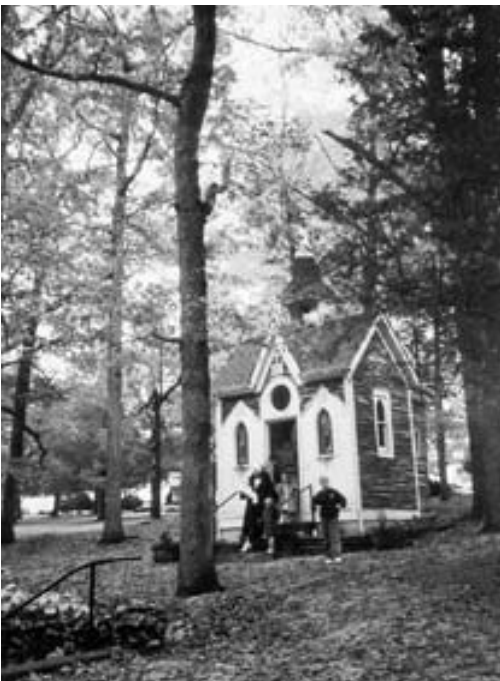
The tiny shrine chapel to Our Lady of Sorrows which was constructed out of logs in 1888, complete with bell tower, stained glass windows and sanctuary apse. The front "walls" on either side of the door, are actually doors which can be opened while Mass is being said to accommodate the view of the faithful kneeling outside and in front of the chapel.
