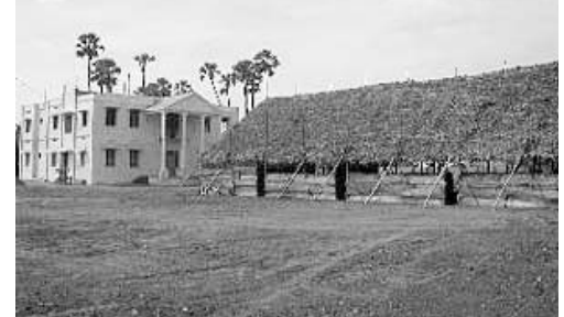
The recently completed “banana basilica” on the grounds of the Society’s complex.
