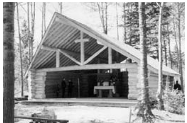
The completed rustic, but prayerful chapel complete with a cross and "M" (for Our Lady) built into the rafters. The chapel is 32 feet by 32 feet, contains a room in the rear for a sacristy as well as enough sanctuary space to accommodate a Pontifical Mass. The land upon which the shrine was built was deeded to the church through the will of a generous benefactor.
