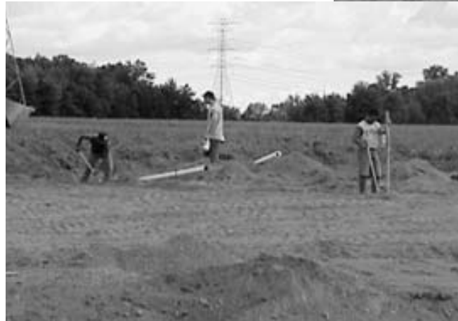
Parishioners work on leech field for new septic system.
