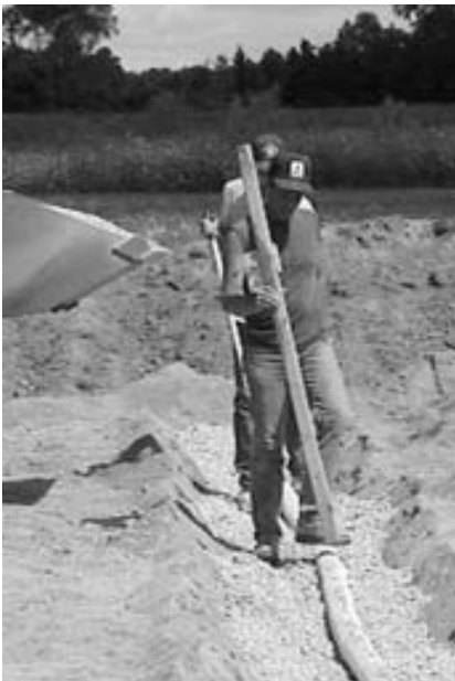
Parishioners work on leech field for new septic system.
