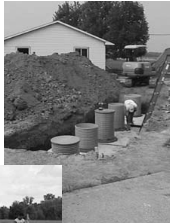
Three new septic tanks are installed as part of the new system.
