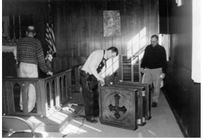
Preparing the communion rail gates for installation.
