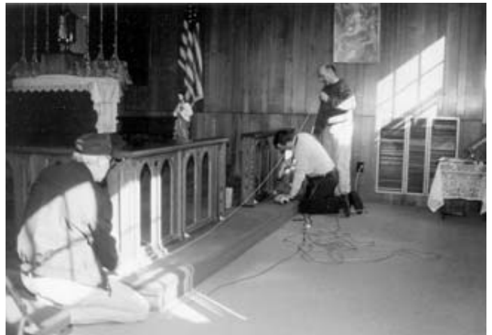
Installing the rail itself.
