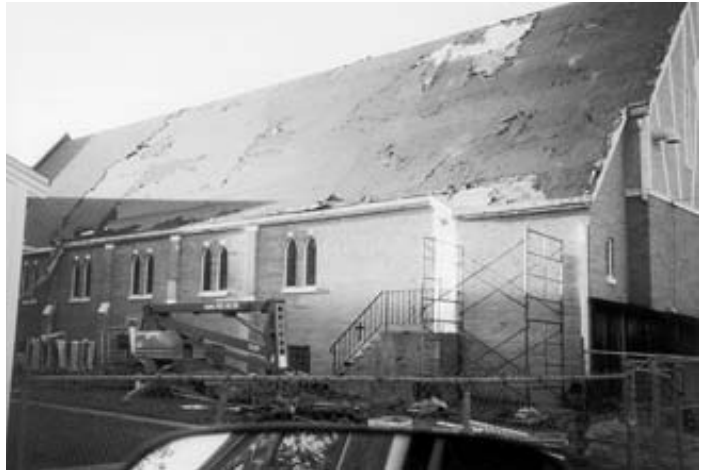
The old shingles were entirely stripped off down to the boards.
