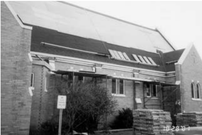
The new shingles were then added on top.
