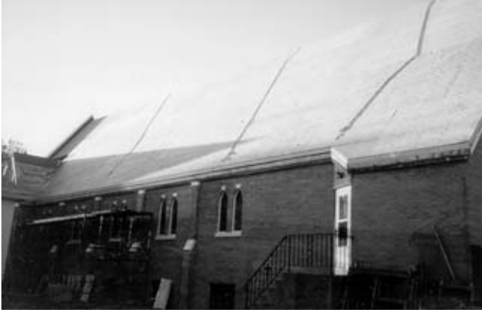
Then insulation was added and secured with plywood.
