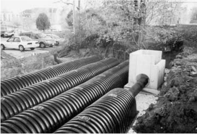
Installing the special drainage system at the bottom end of the parking lot, as required by the city.
