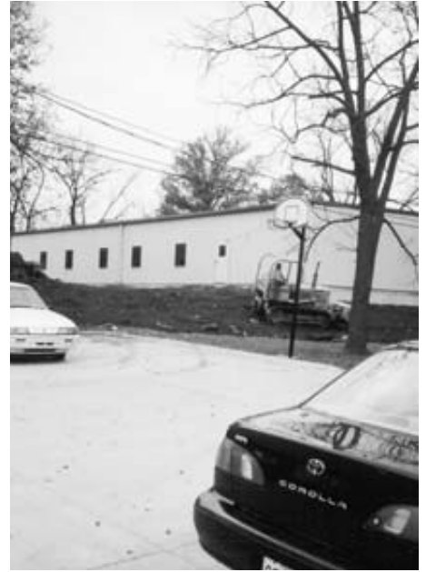
Landscaping over the buried drainage system, as seen from the Regina Coeli House parking lot.
