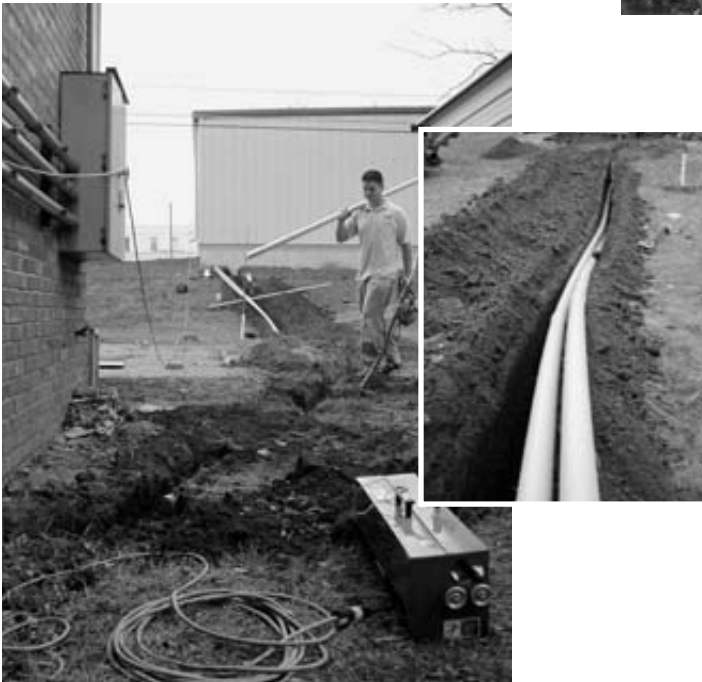
Installing a direct telephone connection between the Regina Coeli House (left), and the Angelus building in the background.
