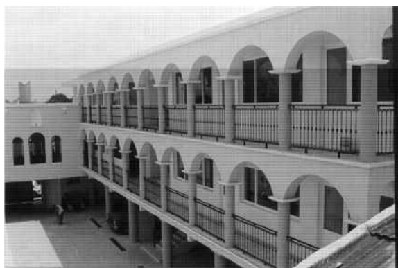
The newly finished school wing at St. Athanasius Priory in Guadalajara.
