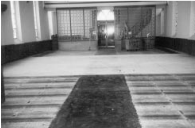
The carpet runner and vinyl tiles are pulled up to reveal the maple floor in need of considerable work.
