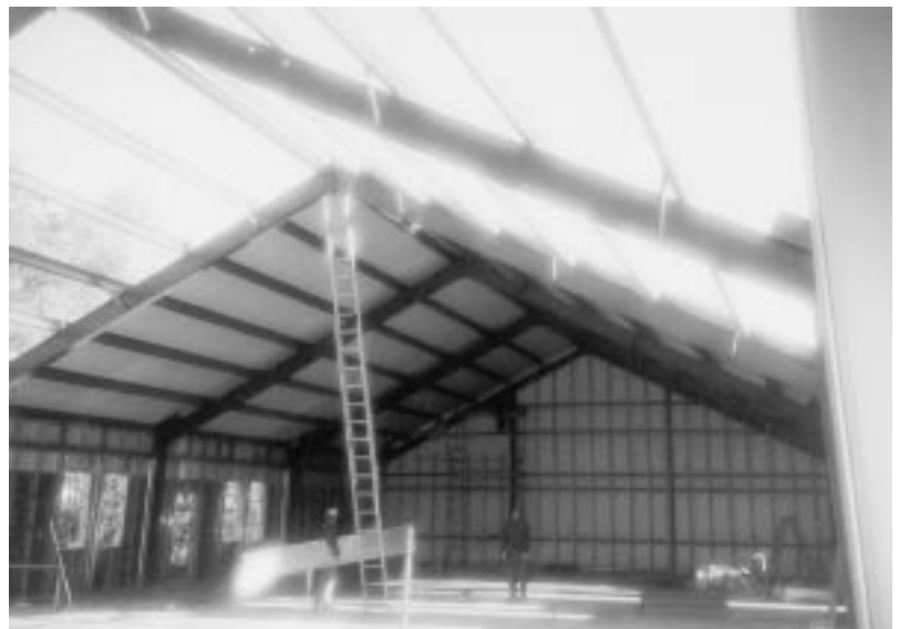
Workers inside the metal building continue work on the exterior structure. The high roof will permit the cathedral ceiling effect, giving the proportions of a church.
