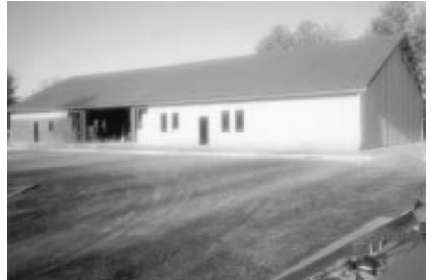
Another side view of the building from the parking lot, but this time from the back.
