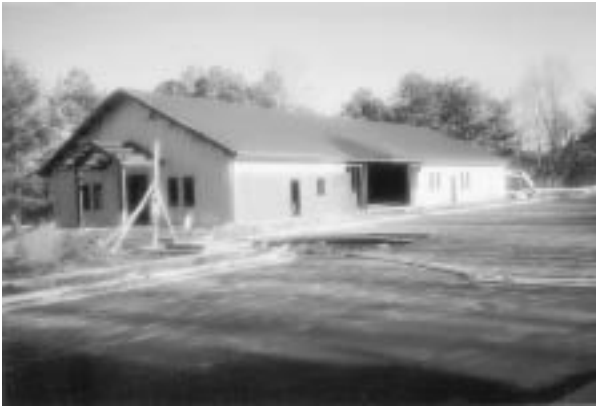
A view of the front and side of the building from the parking lot. The bathrooms, parish hall and kitchen are all in the front half of the building, with the church occupying the back two-thirds.
