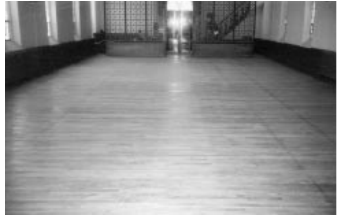
The finished job. Looking back to the main entrance into the church.
