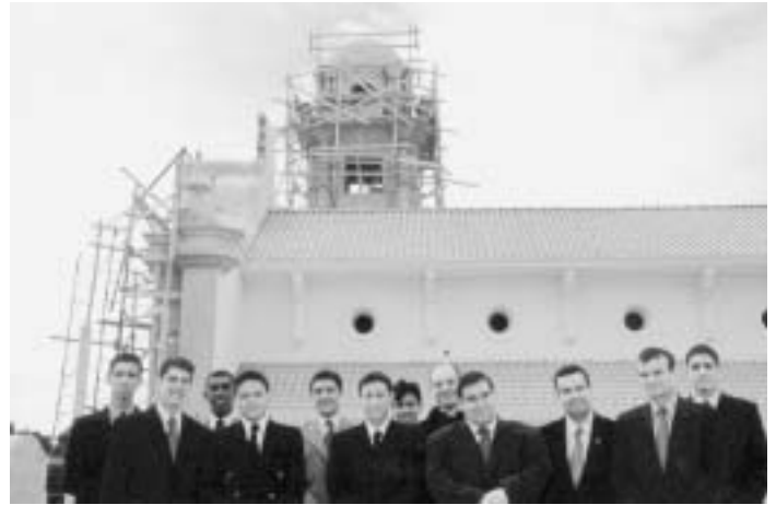
The 12 first year seminarians alongside the new church still in construction.
