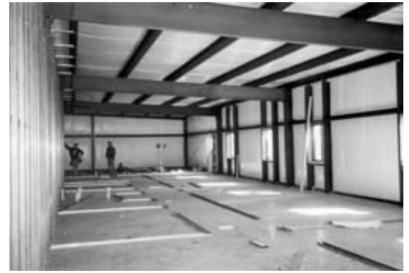
A view of the office area as workers are about to put up the interior walls that divide the different offices.
