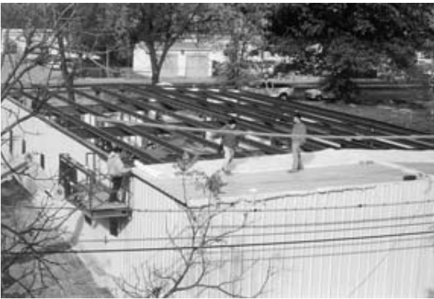
Working on the insulation and roof.
