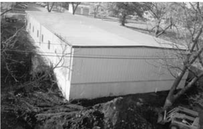
Landscaping around the new building.
