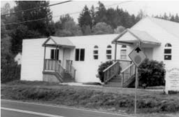
The new main entrance to the humble Our Lady of Fatima church. To the right is the sign and to the left the large flat roof parish hall and classroom addition, just finished last year.
