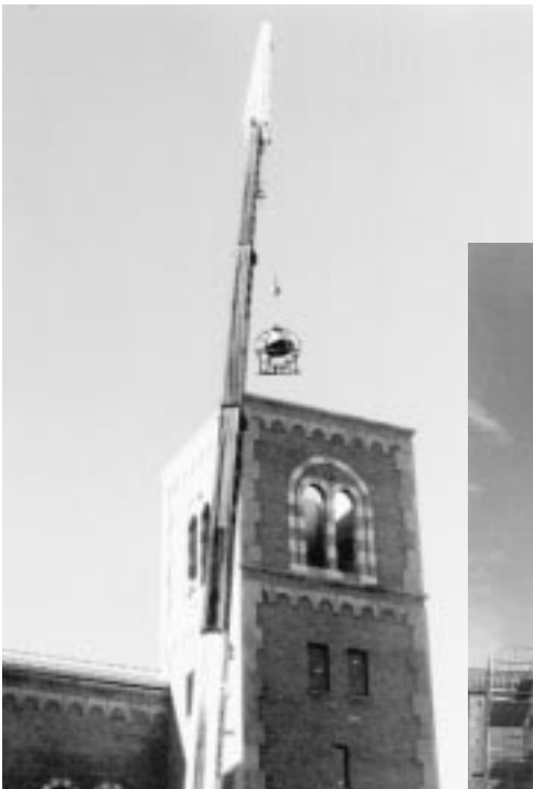
The bell is gently lowered into position in the bell tower.
