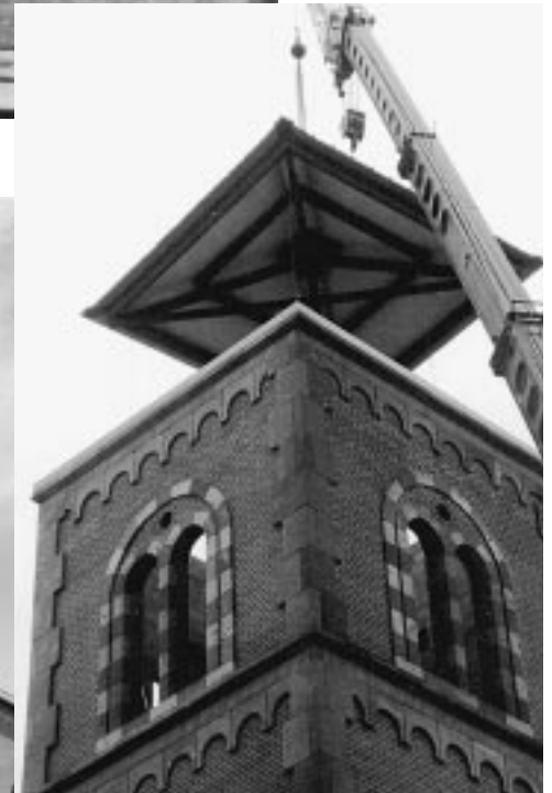
Then the bell tower roof was lowered into position, equally gently.
