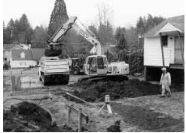
Excavation for the new extension begins, in the quadrangle that used to separate the parish hall and the chapel.
