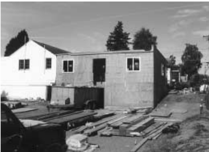
An uphill view of the construction in progress, taken from the parking lot below the parish hall.
