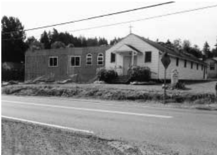
A view from the other side of the road shows the church to the right and the extension to the left.
